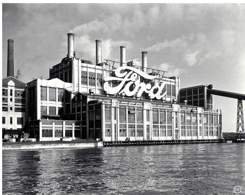
Figure 5 Former Ford powerhouse at Dagenham, Essex Ford developed the idea that generating energy on site greatly reduced costs. Source: Ford Europe
